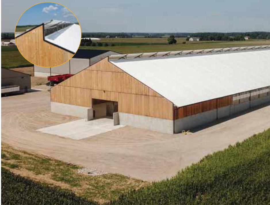
We chose to ventilate with the Overshot Ridge versus chimneys in order to move more air; it has worked very well. **The air is always fresh.**
